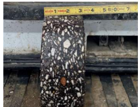
Figure 2 - Runway 10-28 Pavement Core
