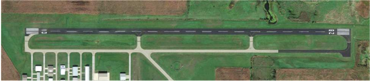
Figure 7 - 2016 Seal Coat Application
