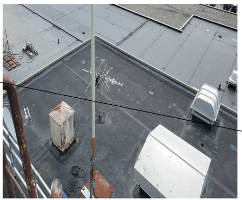
Roof S - Metal deck, 2" ISO, Sm Mod Bit, 2" ISO, FA EPDM
