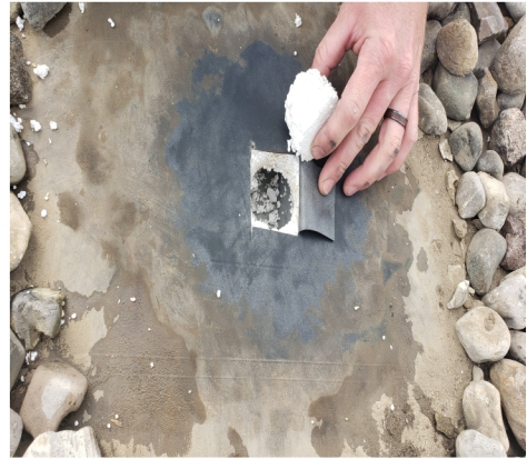
1.5" stone ballast, EPDM, 1.5" EPS, metal deck 20" stretch out coping
