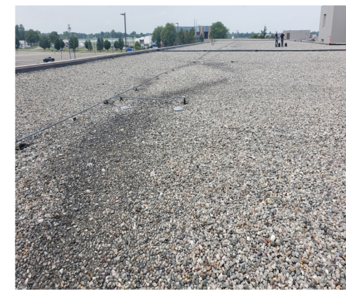
1.5" stone ballast, EPDM, 1.5" EPS, metal deck 20" stretch out coping
